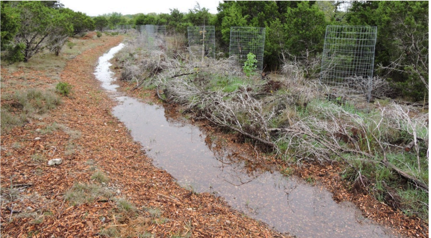
Example of a contour bioswale.
