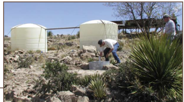
Figure 3. A Black Gap Guzzler rainwater catchment.
